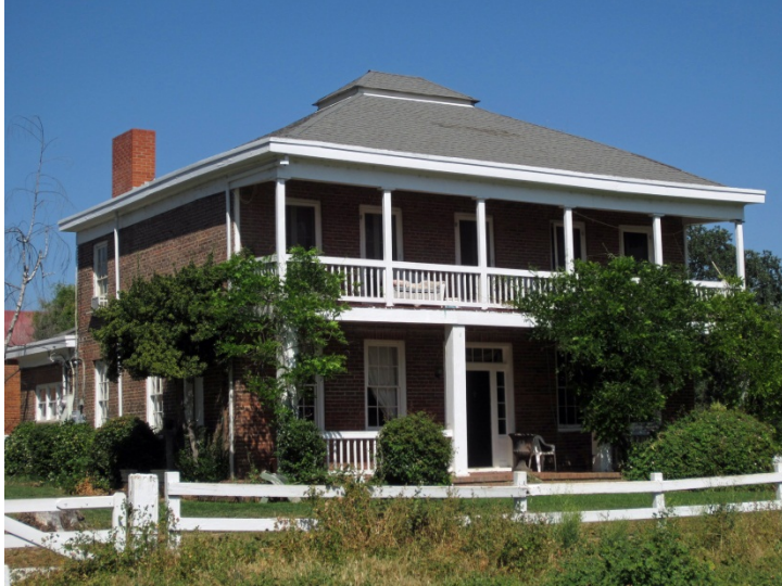
George and Eliza Withington House lone, Amador County
