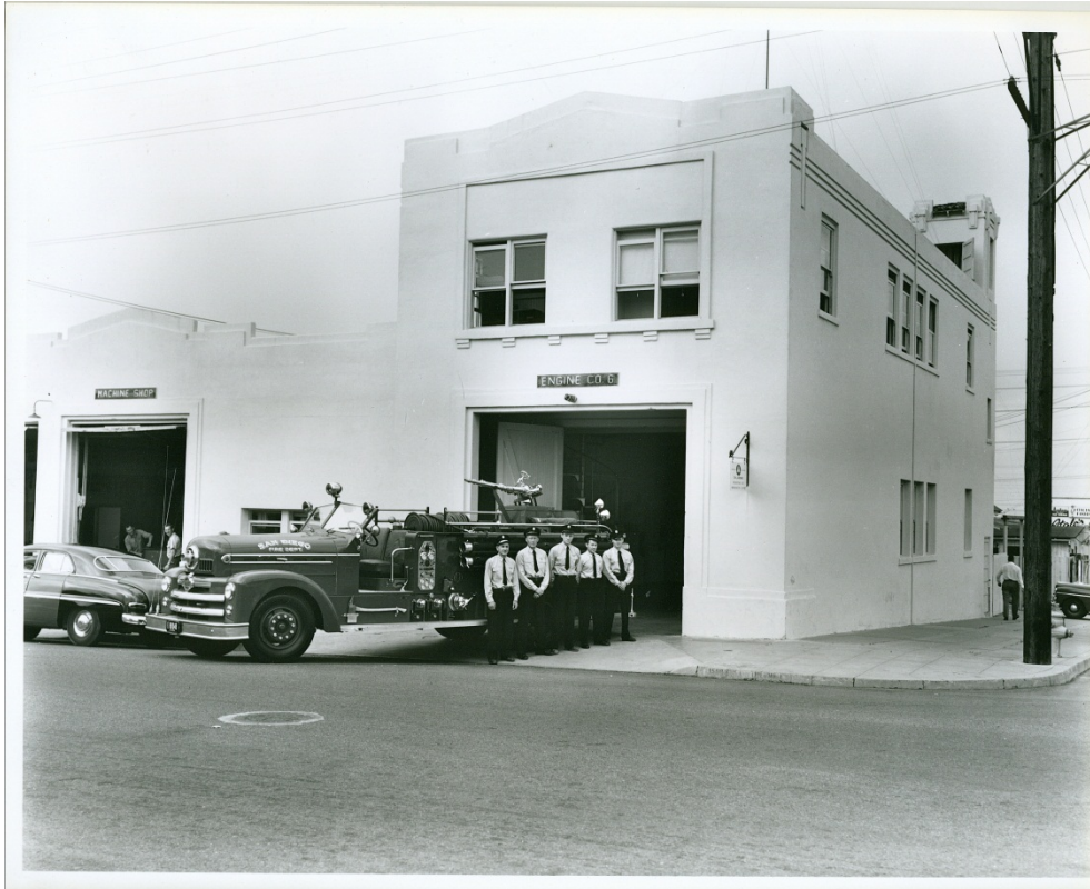
San Diego Fire Department Shops at Station 6 San Diego, San Diego County
